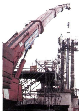
Agen, manutention pylône
