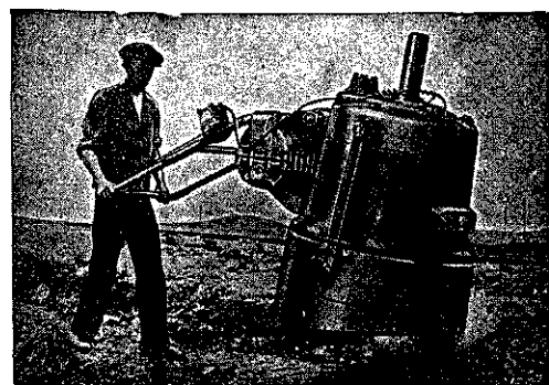
Grenouille DELMAG 1.000 kg Compactage autoroute
